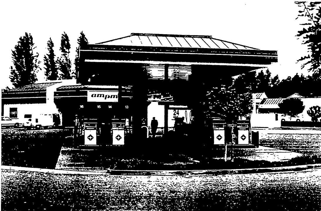
Figure 4.16. View of Fuel Dispension Area in El Toro. This fuel dispension area uses a grading to the center that drains to the curb in front of the planter. Under the planter is a 550 gallon holding tank ( March 24, 1998 ).
