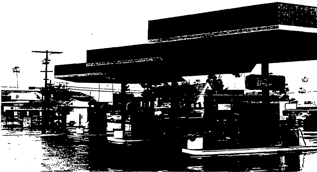
Figure 4.10. Rain canopy in Anaheim. The “zigzag” design of this canopy may be stylish, but it allows way to much direct rainfall on to the fuel dispension area even during mild rainfall events ( February 22, 1998 ).
