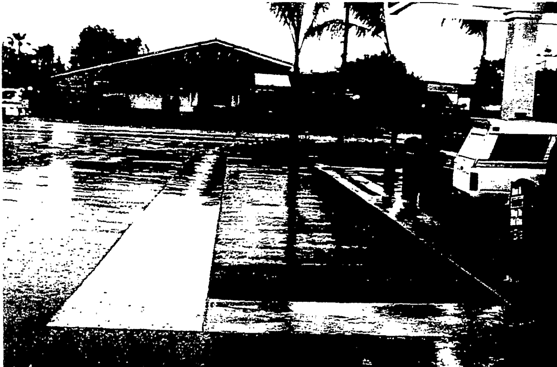
Figure 4.5. Parking lot stormwater gully in Anaheim. This gully collects parking lot runoff and channels it to the street. Even during heavy downpours these channels keep runoff from the surrounding parking lot area from flowing on to the fuel dispensation area ( February 3, 1998 ).
