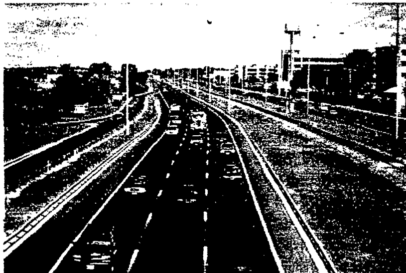
Figure 2.1 Photograph of MoPac at West 35th Street
