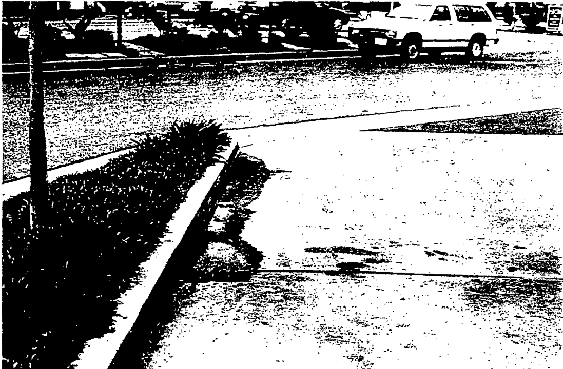
Figure 4.18. Drain leading to underground stormwater storage tank in El Toro. This drain to the 550 gallon tank was always full and overflowing during every stormevent I observed here. There is an access to the tank in the planter that can be used to pump out contaminated water. ( March 24, 1998).
