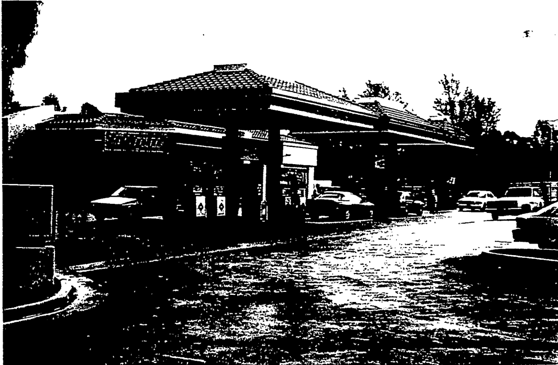
Figure 4.12. Rain canopy in Laguna Hills. This 3 stage canopy design contains more surface area on its sides than a single rectangular type, thus the fuel dispensing area receives more stormwater in the form of drippings. Its narrow design also allows more rainfall even at the slightest slant to penetrate deep in to the fuel dispensing area ( March 4, 1998 ).
